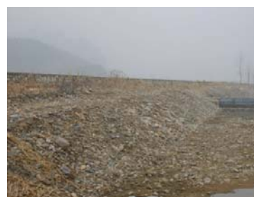
Figure 1. Experimental area before soil bioengineering construction in Huaijiu River
